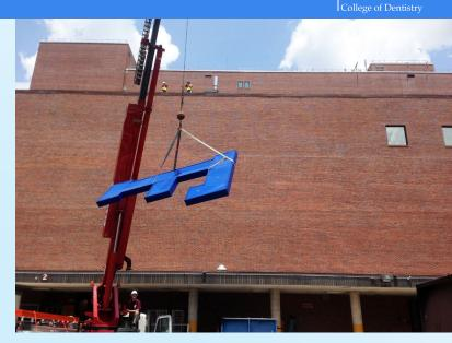
The parts of the new UF College of Dentistry sign were lifted by crane onto the roof over the third floor of the tower. Crews erected scaffolding and are assembling the pieces to create a new sign on the west wall of the dental tower's 11th floor. The work is expected to be completed by July 1.
